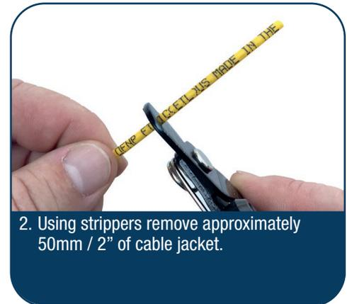
2. Using strippers remove approximately 50mm / 2" of cable jacket.
