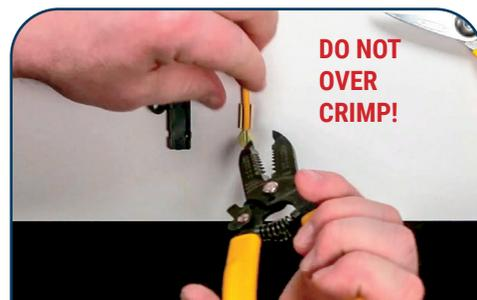
6. Place the brass jacket crimp under the cable flush with the end of the cable jacket. Use pliers to bend the jacket crimp just enough so that it holds the cable jacket.
