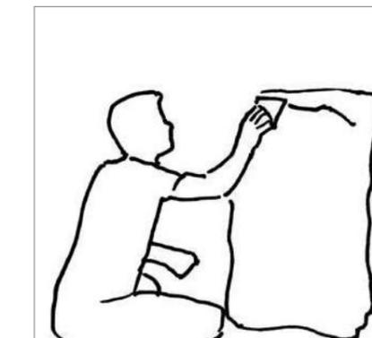
Up to 2mm of plaster can be applied, thus, Q3 and Q4 wall /ceiling quality levels are easily possible.
