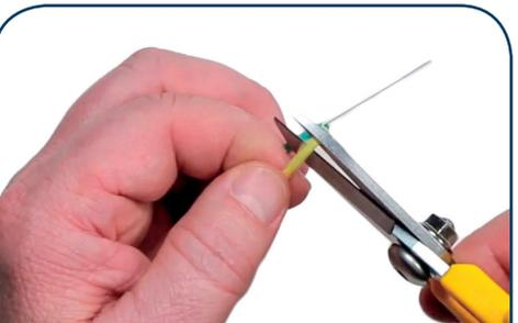
6. Hold the aramid yarns back and locate SSF fiber. Trim the yarns closely to the jacket.
