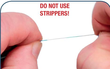
7. Using only fingertips/nails remove Soft Peel 250 μm coating completely from the fiber to within approximately 12 mm or 1/2" of the cable jacket. Repeat process for other cable.
